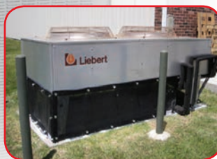
DRY COOLER INTAKE FILTERS
