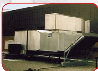
AIR HANDLING UNIT INTAKE FILTERS
