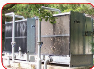
COOLING TOWER INTAKE FILTERS
