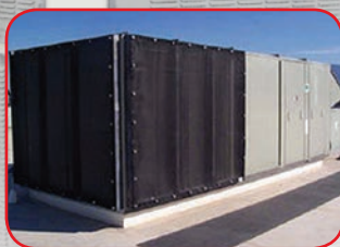
ROOFTOP UNIT INTAKE FILTERS
