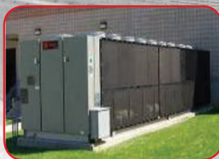
CHILLER COIL INTAKE FILTERS
